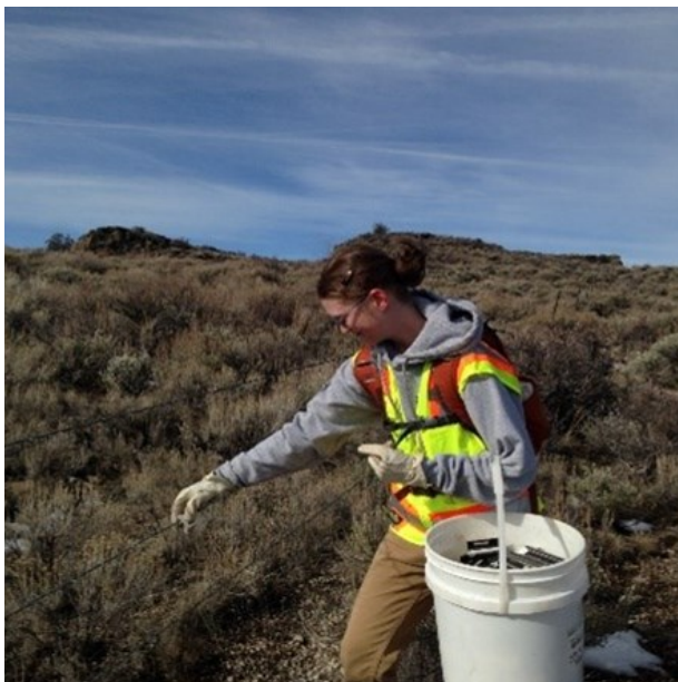
HOC AmeriCorps crews repaired range fencing located to the east of Bend. Updating old fencing improves wildlife migration, while protecting threatened and endangered species. Amber, a Land Stewardship Trainer, exhibits how to place reflectors on the wire fence.
